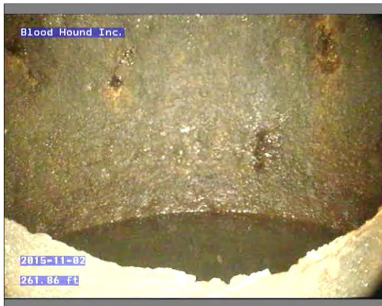
Photo: 45639-110215-01-AECOM-10211201512085712085757_A.JPG, 00:29:32 262FT, End of Pipe
