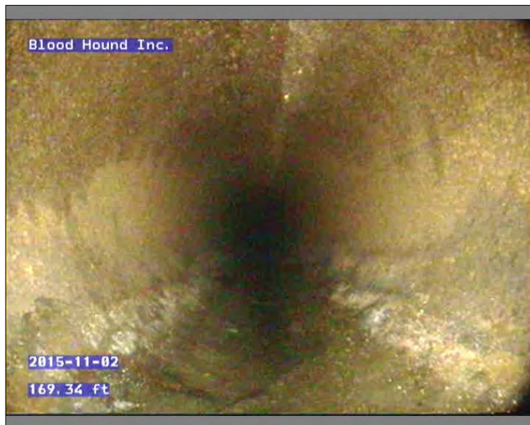
Photo: 45639-110215-01-AECOM-10211201511582111582121_B.JPG, 00:21:26 169.34FT, Material Change, Steel pipe
