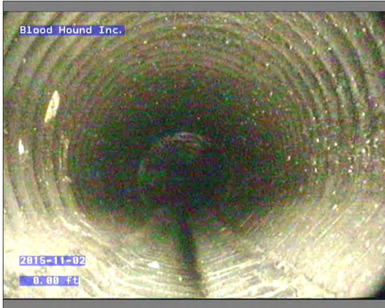
Photo: 45639-110215-01-AECOM-10211201511312111312121_A.JPG, 00:00:00 0FT, Discharge Point
