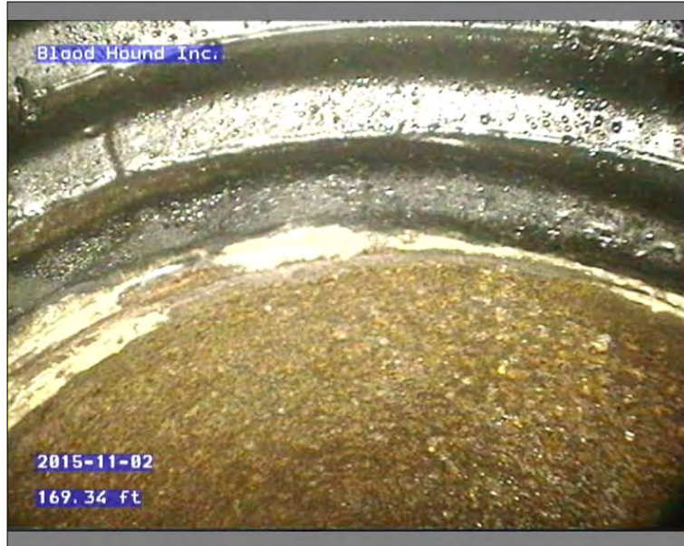
Photo: 45639-110215-01-AECOM-10211201511581211581212_A.JPG, 00:21:26 169.34FT, Material Change, Steel pipe
